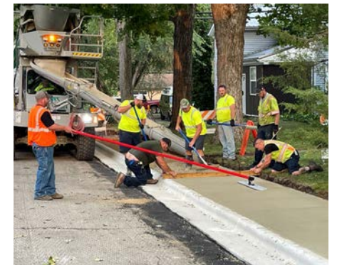
High quality trail construction and regular maintenance practices are essential to encouraging use of the system.
