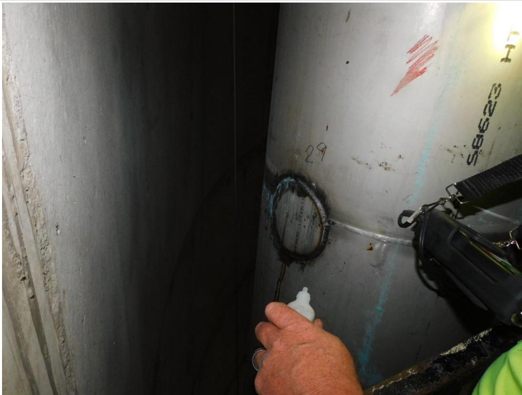
Photograph #: 7 Date: September 2, 2025 Subject: Previous Inlet/Outlet Pipe Patch Repair ('87 feet)
