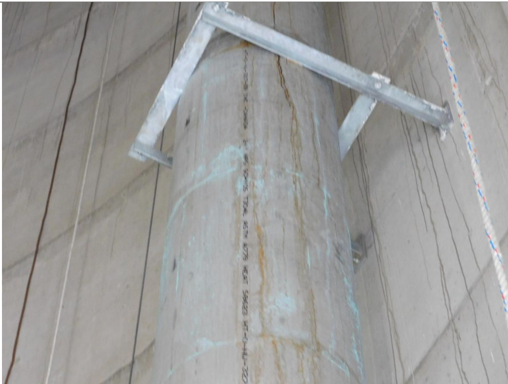
Photograph #: 4 Date: September 2, 2025 Subject: Inlet/Outlet Pipe Support (Typical)
