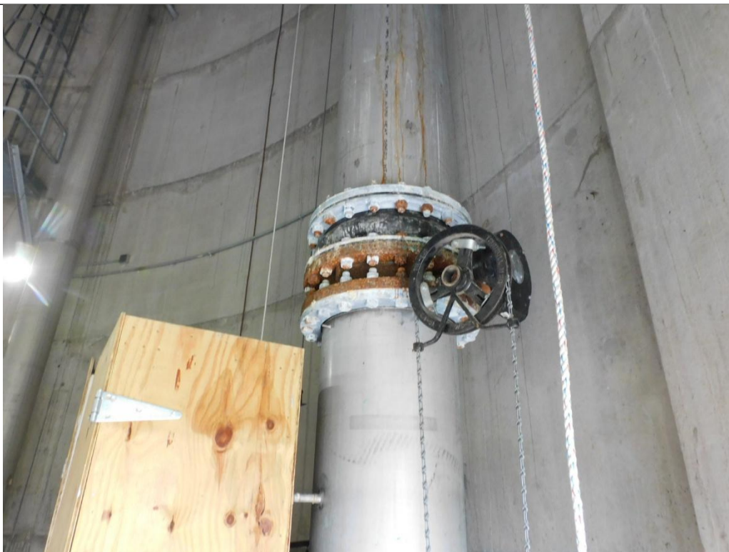
Photograph #: 2 Date: September 2, 2025 Subject: Expansion Joint and Butterfly Valve
