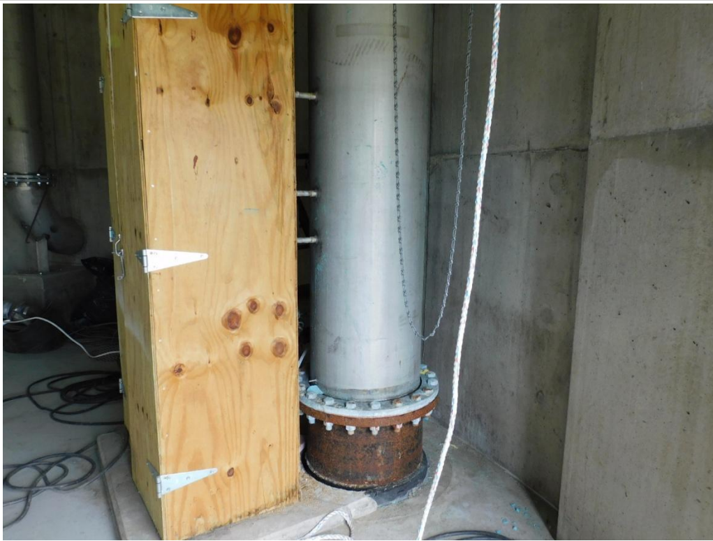
Photograph #: 1 Date: September 2, 2025 Subject: Inlet/Outlet Pipe at Tower Base
