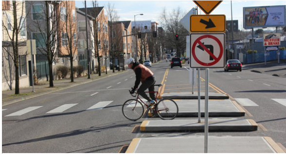
Median Refuge Island
