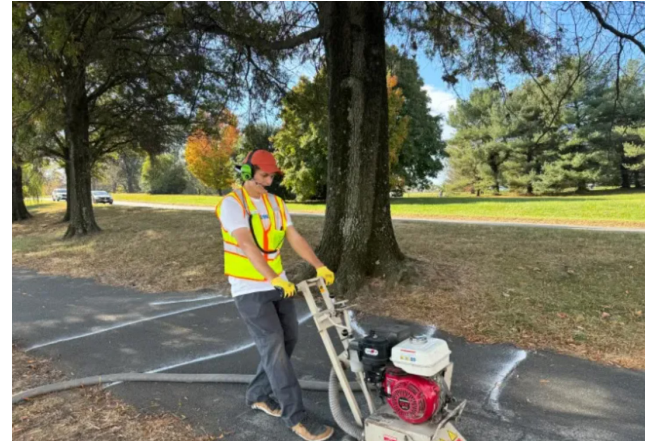
Trail maintenance to improve trail surfacing
