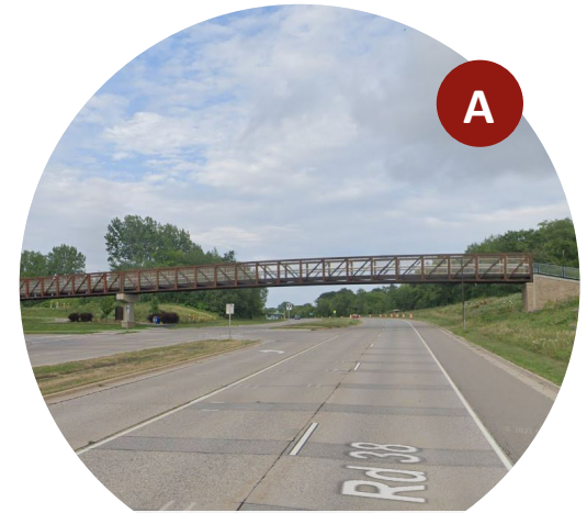
Pedestrian Bridge over County Road 38, part of RBTN Alignment
