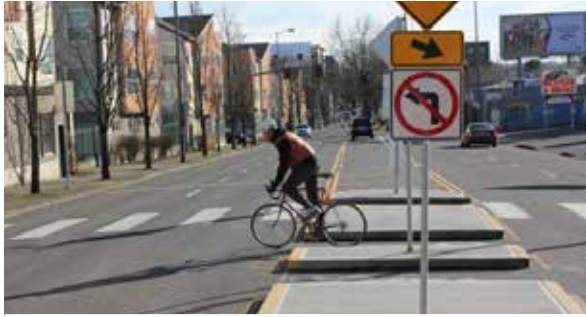
Median Refuge Island
