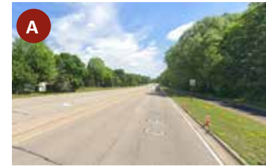
Looking west along CR38, there is a trail gap on the south side of the road.
