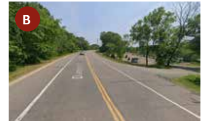
CR 33/Diamond Path has identified trail gaps on both sides of the road.
