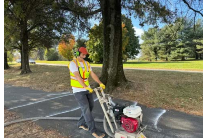
Trail maintenance to improve trail surfacing
