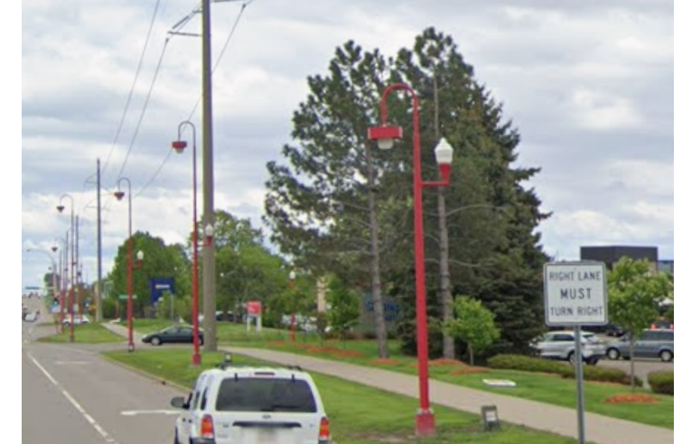
Existing Overhead Power and Lighting (Gleason Path & CSAH 42)
