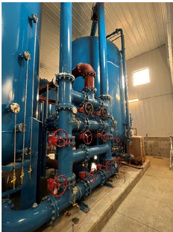
Figure 2-6. GAC Unit and Valve Arrangement
