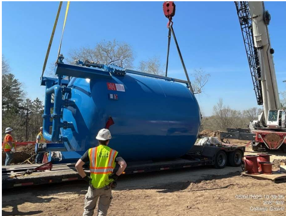
Figure 2-3. Installation of GAC Vessel
